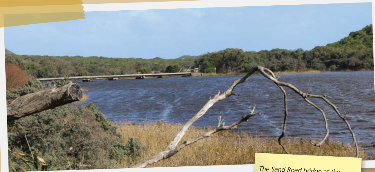
The Sand Road bridge at the Aire River estuary
