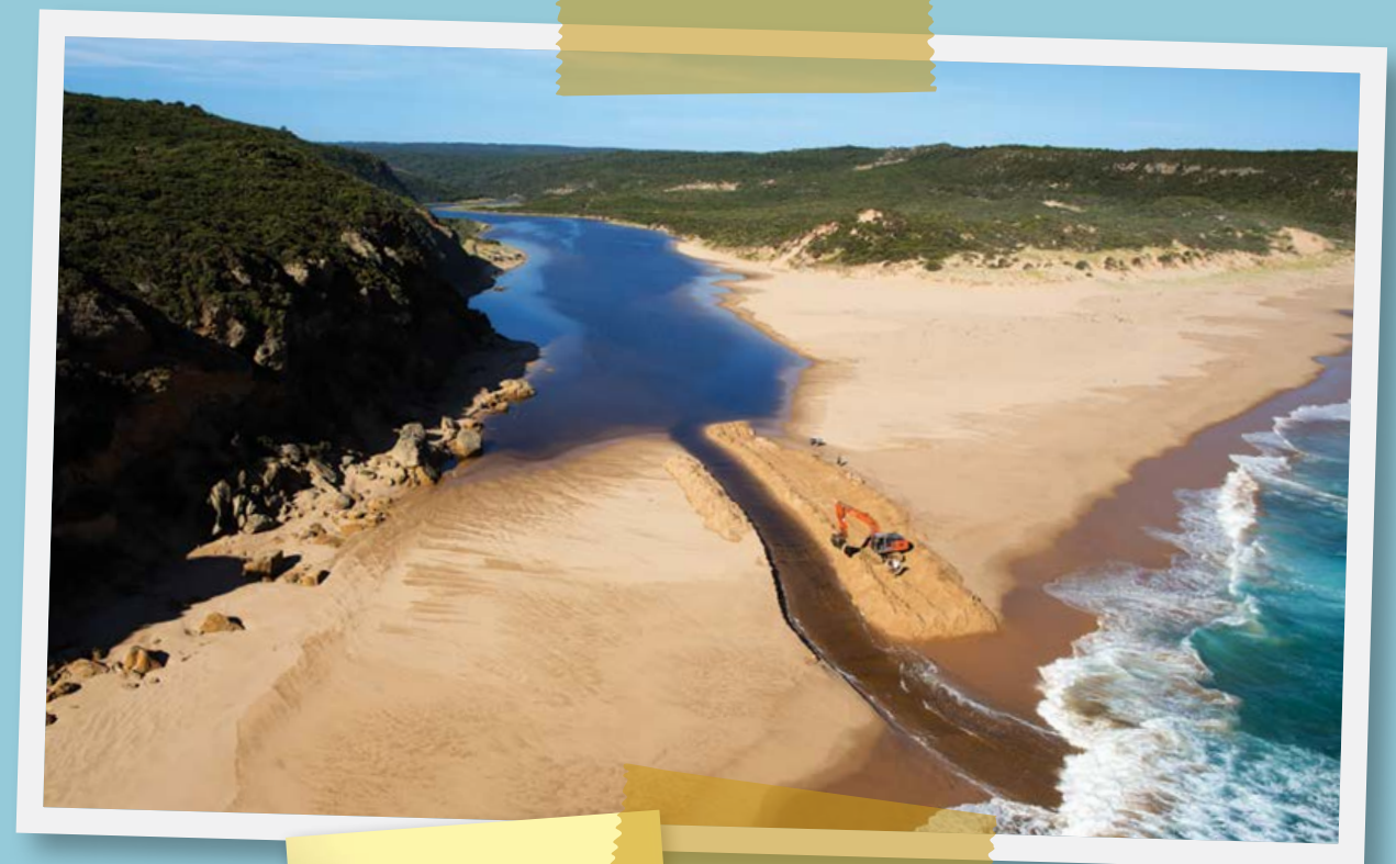
Artificial opening at the Aire River estuary
